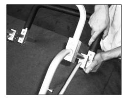
2.1 Fit the lower rear crossbar (C) to the left and right side arm assemblies (A).
